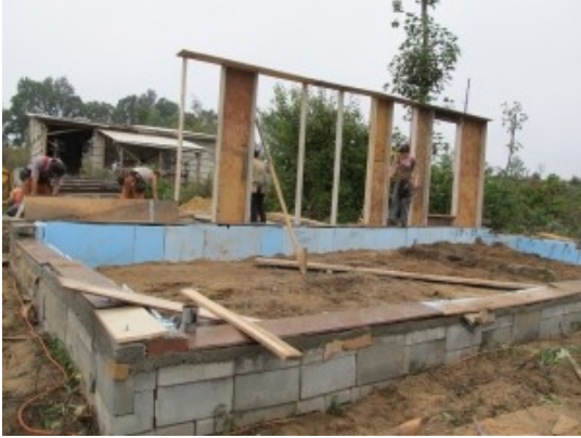
Framing the first wall of the greenhouse.
